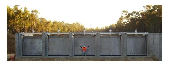
Goulburn-Murray Water: Measure, design, construct and install 80 fully automated gates including software and integration into TCC SCADA system for the Strategic Measurement program. Also design, construct and installation of over one hundred automated channel systems throughout G-MW's areas of operation (LEVTROL).
