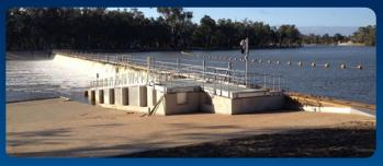
Mildura Weir's new gates eliminate all OH&S issues associated with the insertion and removal of timber drop bars and provide improved regulation and isolation capacity.
