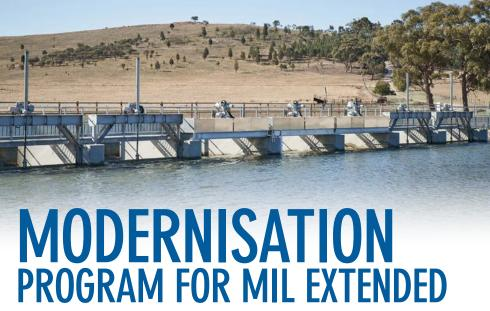
AWMA have successfully delivered 55 water control gates for Murray Irrigation's 'PIIOP Round 3' which substantially increased water efficiencies, enabled ordering flexibility and significantly reduced leakage through infrastructure upgrades. These works included 12 Mulwala Canal sites (28 LayFlats and 20 Undershots), Lawson Syphons (two Undershots), the Edward River Escape (two Bulkhead gates) and the Wakool Canal Offtake (three Undershots).
