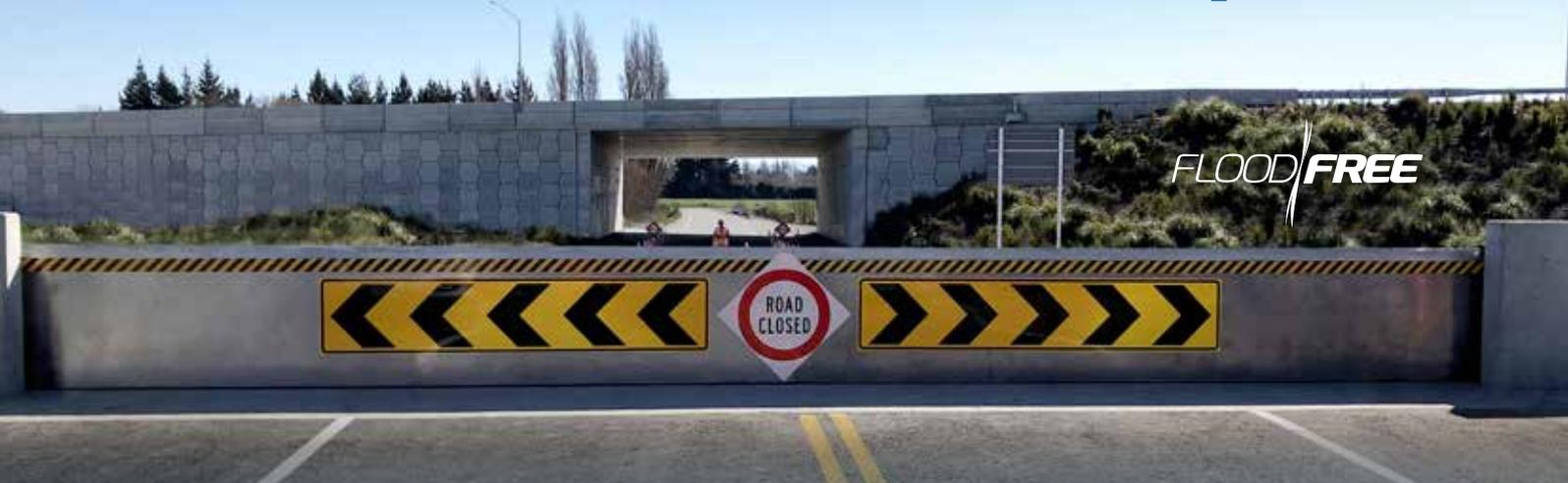
**A FloodFree Retractable Flood Barrier was exported to New Zealand and installed at Dickeys Road, Belfast, to complete the secondary flood protection system for Christchurch. The Flood Barrier was needed to contain a large (6500 cubic metres per second) design flood in the Waimakariri River.**
