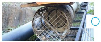
Installing a coarse screen
