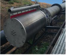
Before (left) and after (right): coarse pump intake screen replaced with AWMA Self-Cleaning Intake Screen.
