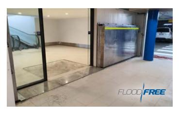
Covers located on the track system and end panel protect the infrastructure when not in use, but are easily removed in emergency situations.
