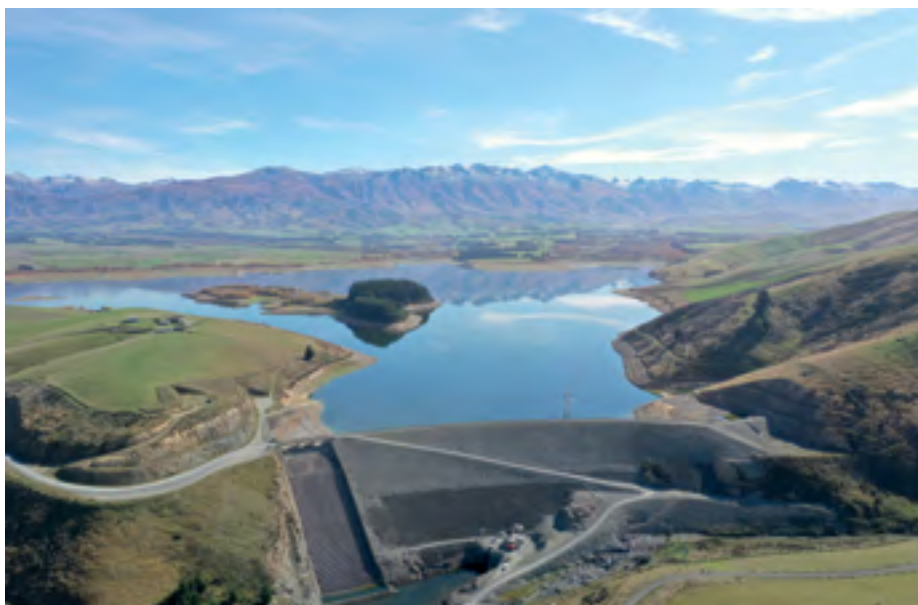
The Opuha Dam and Lake – which showed its adaptability during dry conditions in early 2021 and also incredibly high rainfall come May.
