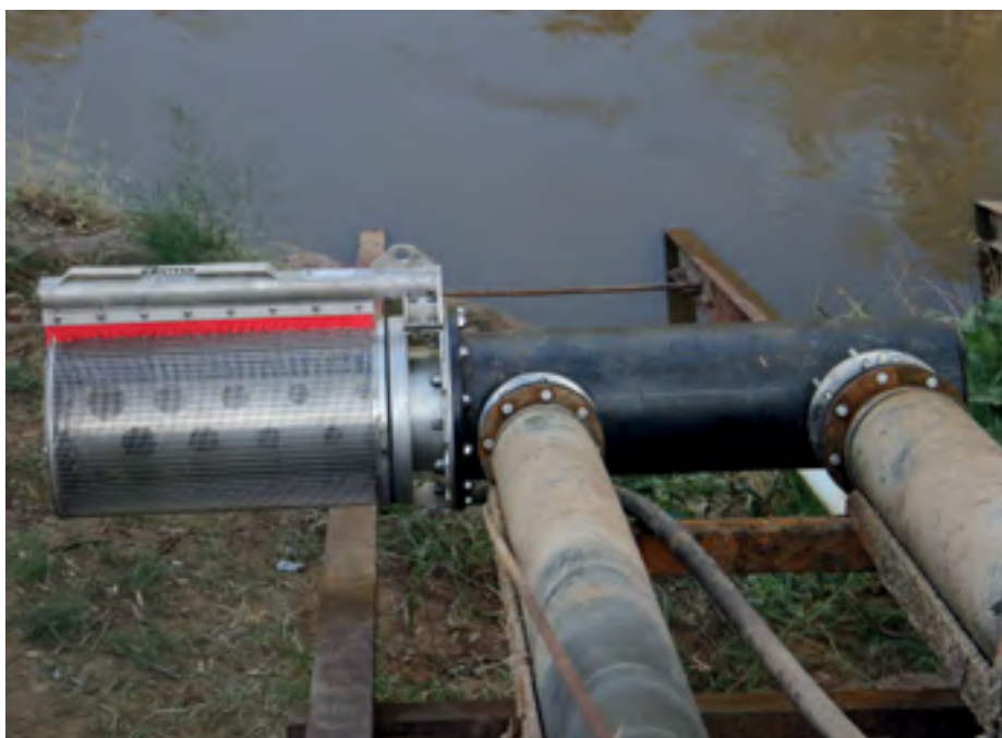
Cylinder screen on dual pipe.
