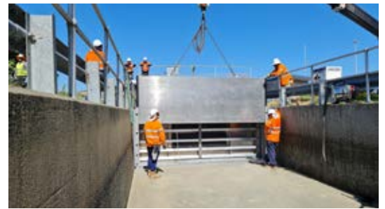
Left- Completed Concealed Flood Barrier Right- Concealed Flood Barrier during installation
