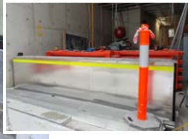
Left- Completed Concealed Flood Barrier Right- Concealed Flood Barrier during installation
