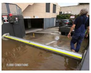
^ Pictured above is the FloodFree Passive Tilting Flood Barrier which self-deploys as water levels rise.
