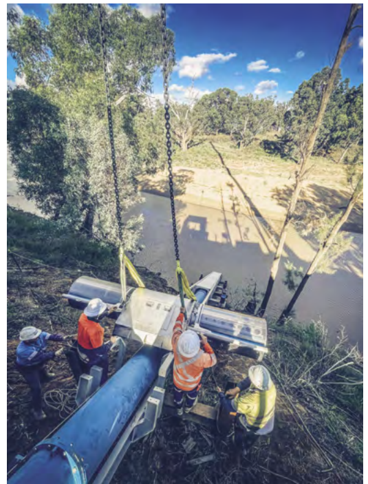
The high-tech, modern screens are retractable, so can be moved out of floods and serviced more easily.
