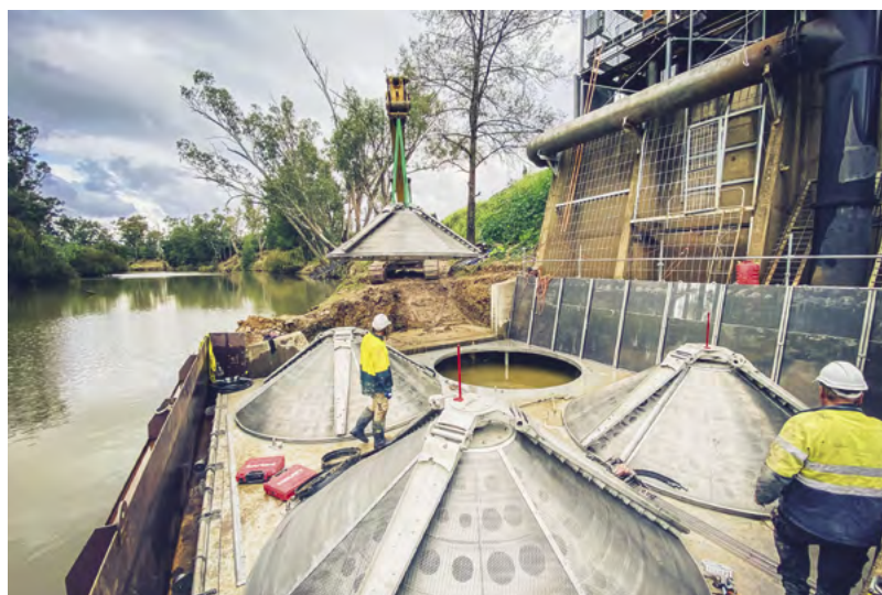
ABOVE: Four, self-cleaning cone screens being fitted to the Trangie-Nevertire Irrigation Scheme main pump.
