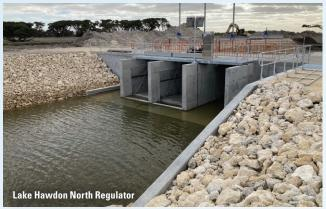
To maintain aquatic connectivity, one fishway gate remains open during regulation periods, enabling upstream fish passage. During high-flow periods in winter, the structure allows for passive discharge, reducing flood risk, while isolation gates enable controlled diversion over the LayFlat regulators as seasonal conditions shift.
