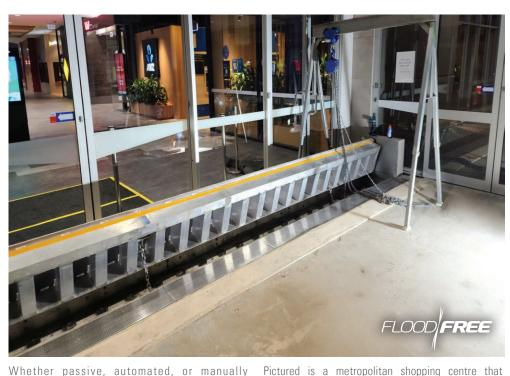
Whether passive, automated, or manually operated, AWMA designs prioritise practical performance, end-user functionality, safety and operational preferences. Key design considerations include high traffic loads, emergency access, backups, manual overrides, integrated alarm systems, fast deployment and reset capabilities to minimise downtime post flood event.
