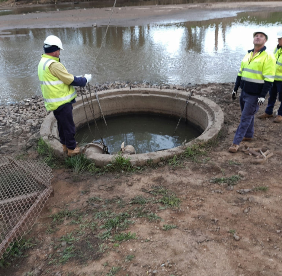
REPLACED ORIGINAL SCREEN PRONE TO BLOCKING
