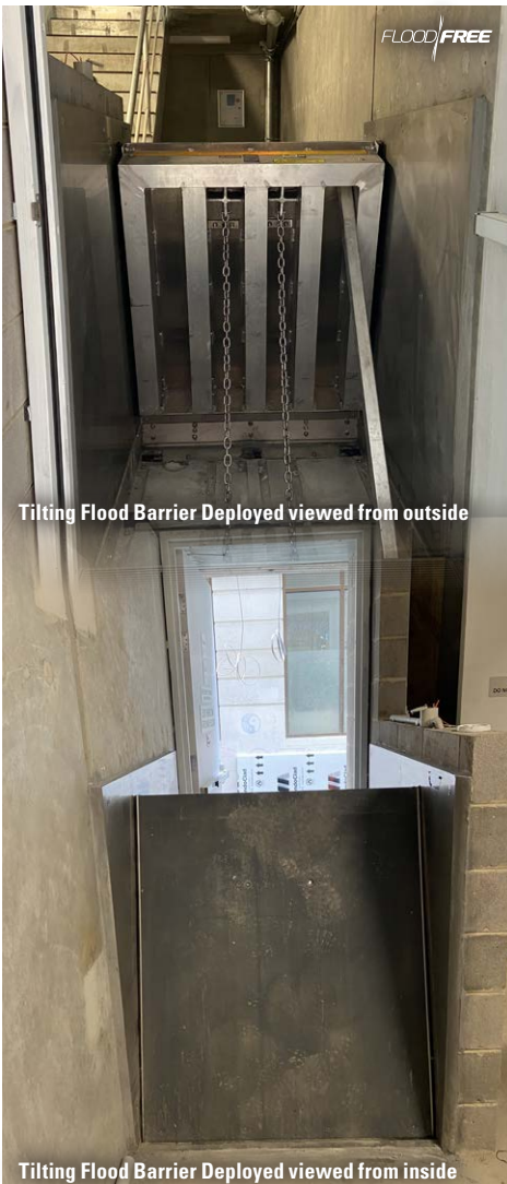
Tilting Flood Barrier Deployed viewed from inside
