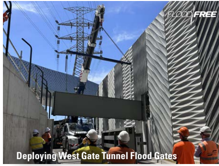
West Gate Tunnel Flood Gates Installed
