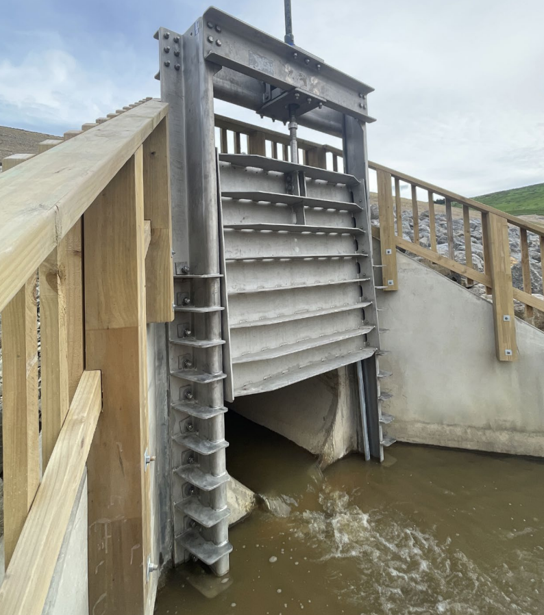
Gate installation for the Koondrook-Perricoota Forest Project's levee at Shear Paddock (Photo courtesy of the NSW Department of Climate Change, Energy, the Environment and Water)
